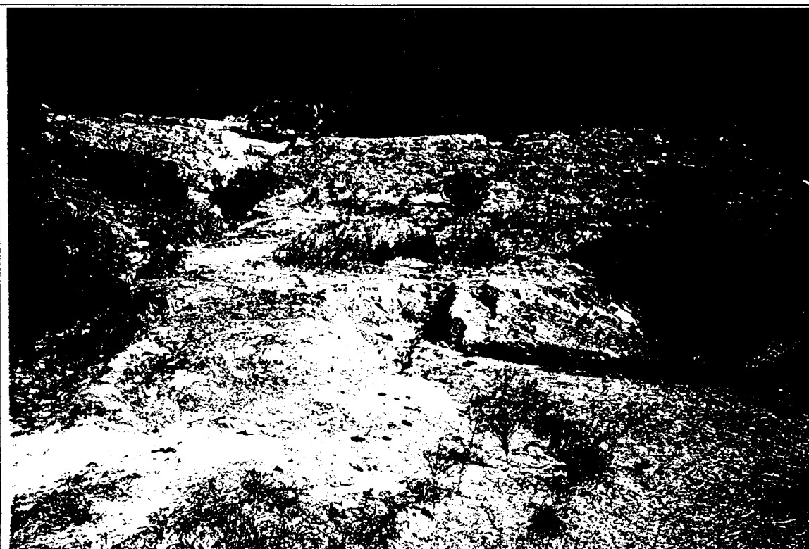
Photo 6-12: Eroded downstream face of the dam south of Buena Vista Mine on the Klau Branch of Las Tablas Creek (10/7/92).
