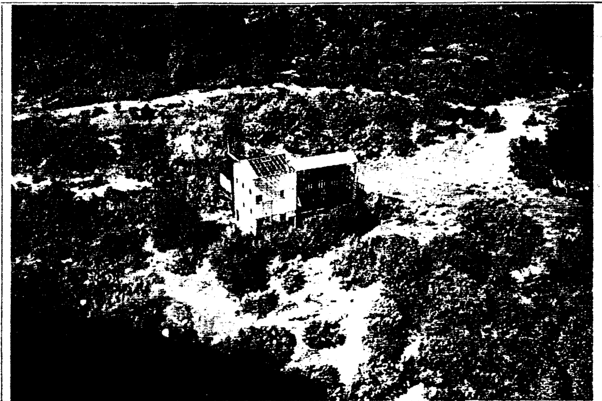
Photo 3-4: Abandoned processing buildings at the Ocean View Mine showing the condenser facility at the right (3/16/92).
