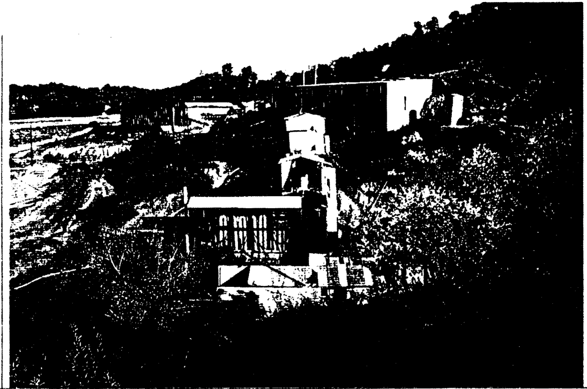
Photo 3-3: Abandoned processing buildings at the Buena Vista Mine showing the condenser facility in the foreground (12/10/91).
