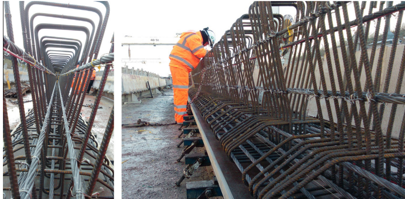
Fig. 2. Installation of fibre optic sensors on beam reinforcing cages.
