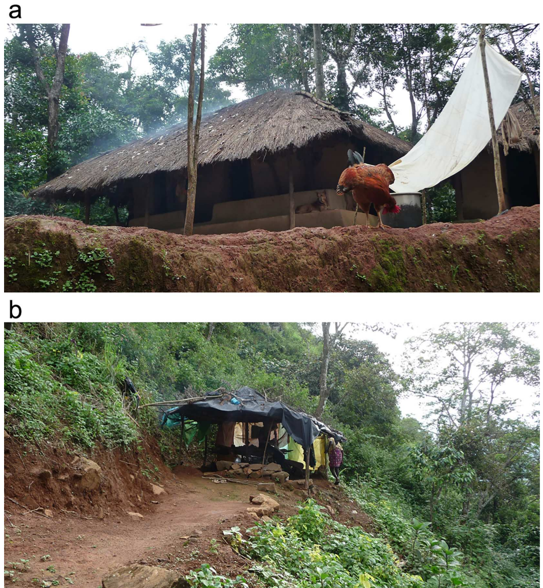
Fig 3. Typical Nayaka houses. (a) A house located on a flat terrace which ends in a steep slope. The house is built on a platform made of stones and mud. Walls are partially made of mudbricks, branches, bamboo and grass and in some cases plastered with mud. The roof is made from branches covered with grasses. Note how the roof extends the house outline leaving the edges of the platform to be used as an open, yet roofed, veranda; (b) A typical open house. The house lack walls and while the structure is made of branches the roof was made of plastic sheets. Note how the house is located on a terrace made by incision in the forest steep hill slope.
