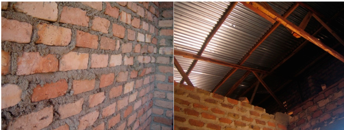
Figure 5. Brick walling and iron sheet roofing is the prevailing construction method in Uganda.
