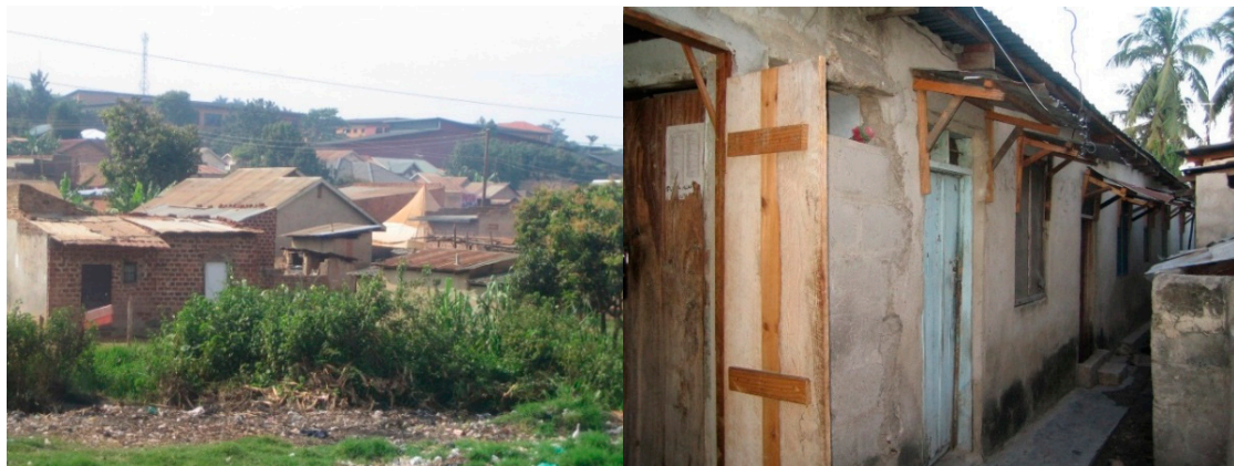
Figure 1. Low-income housing and slums.
