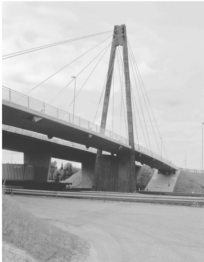
Figure 2 – Photo of Herning Footbridge ( Courtesy of COWI Consulting Engineers )
