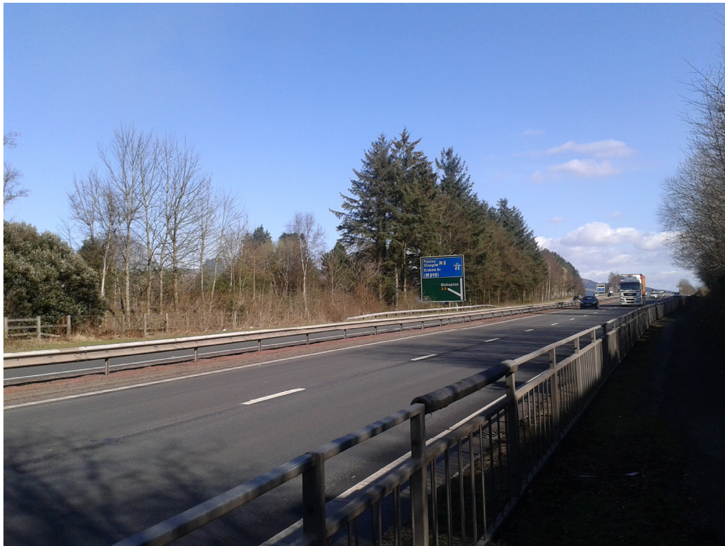
Figure 2. The road to Glasgow.
