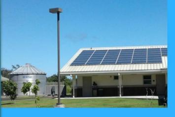
Good "active" design: Photo-voltaic panels turn sunlight into energy to power library systems. Catchment tank stores water for flushing toilets. Cost-high, but pays off in the long run.
