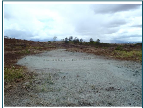
A grassed waterway used to stop gully formation on an individual farm will be more effective and less likely to wash out if it is part of an area-wide effort within a drainage to absorb more rainfall and reduce runoff.
