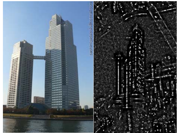
Fig. 7: St. Luke's Tower in Tokyo; left: photo of the building; right: SCR estimation on the building showing the point scatterers (resolution: 1m x 0.6m)
