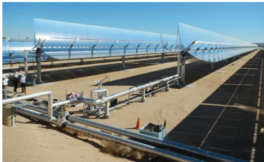
HelioTrough in US with workers
