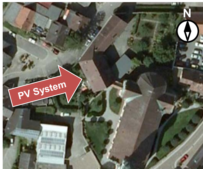
Figure 1: Location and orientation of the PV system used for BEV charging
