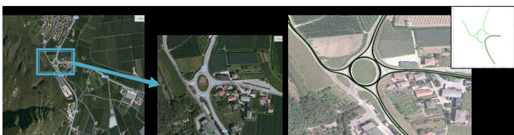
Figure 15.5: Satellite image of the Romagnano roundabout (taken from (11)) and data acquired for its detailed mapping
