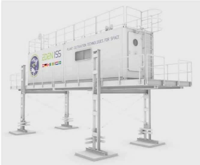
Figure 6. Illustrative impression of the EDEN ISS Mobile Test Facility mounted on the elevated platform (note that the image shows the complete platform, the bottom half of the pillars will be buried in the Antarctic ice) (Credit: Lquifer Systems Group).
