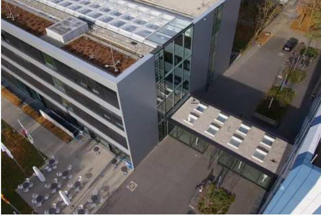
Figure 5: Target building of the EOC-UAV aerial and indoor datasets.
