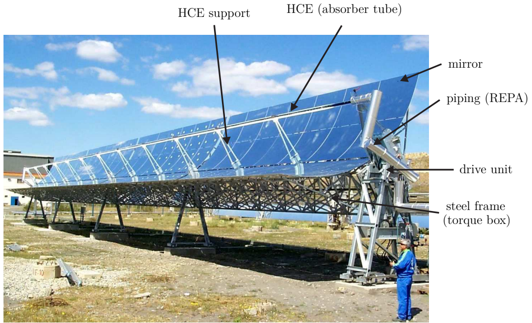
Figure 2.10: (Four) EuroTrough Solar Collector Element(s) (SCE) (cf. [9])
