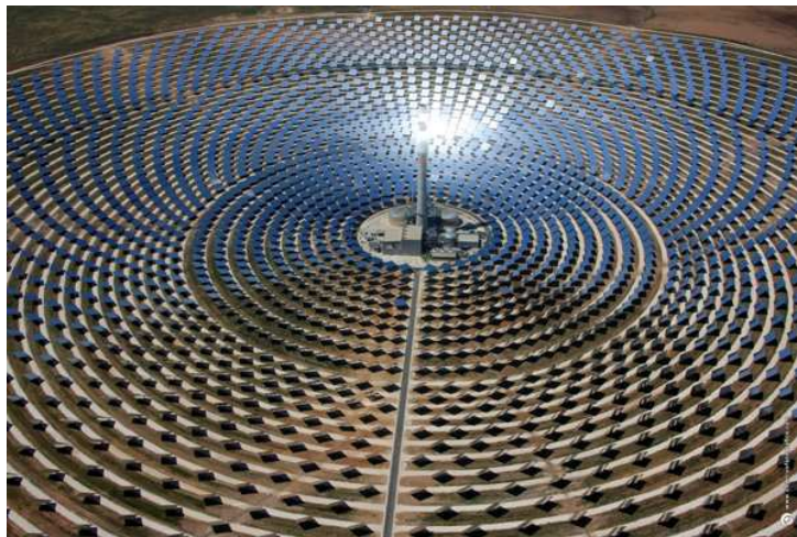
Figure 2.5: Areal view of the Gemasolar power plant surrounded by a 360^\circ solar field consisting of 2.650 heliostats (Photo: Torresol Energy ) [10]
