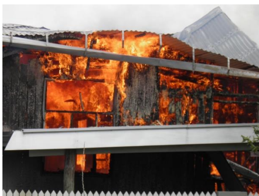
Figure 1: A recent property fire incident in Suva
