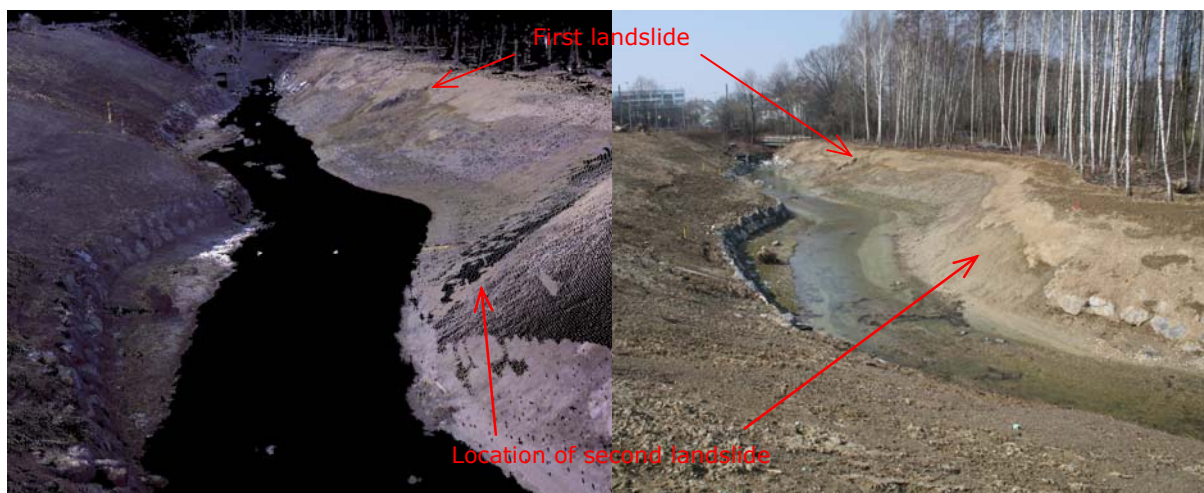
Figure 1: Views of the Sorge River to the West (taken on March 16 th 2006). The point cloud of the laser scanner and the photograph show the area of the remedial works that were done in 2005. The scar of the first landslide is also shown.
