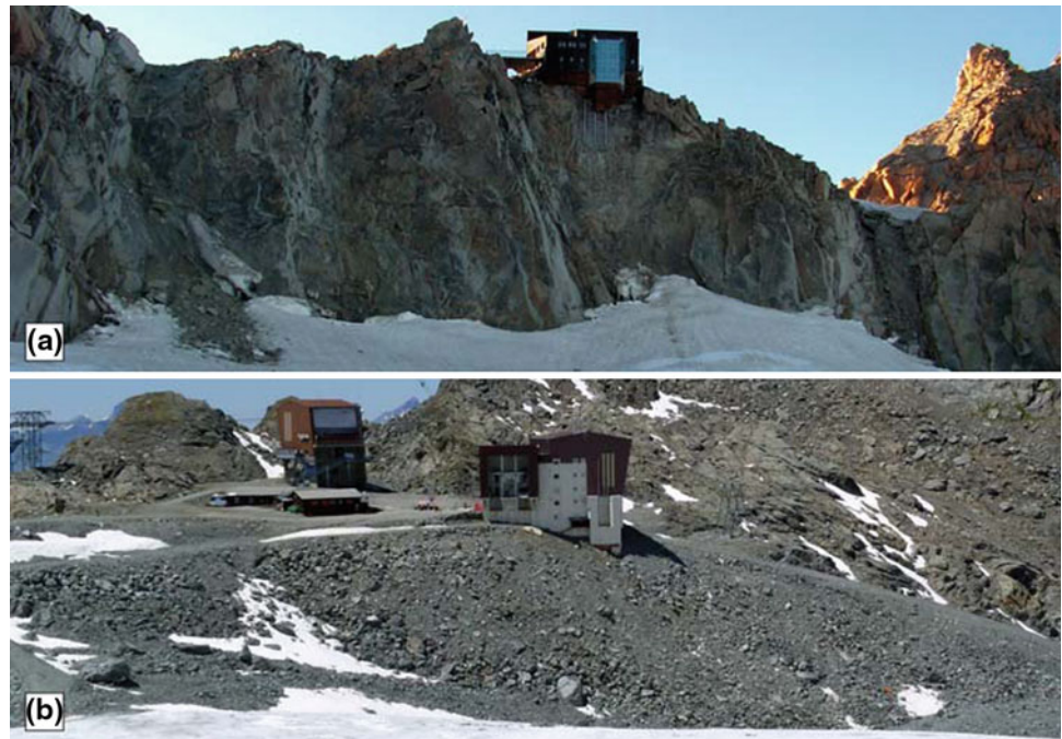
Fig. 32.1 a The lower Arête des Cosmiques with the Cosmiques hut (3613 m a.s.l.) on it; b the inner side of the Gentianes moraine (2894 m a.s.l.) with its lower Mont Fort cable-car station
