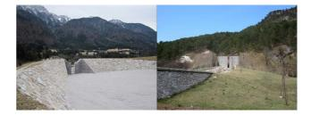
Figure 6. Structural debris flow mitigation measures in Malborghetto-Valbruna, Italy.
