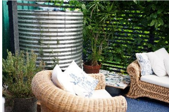
6C(i): Rainwater system – tank.
