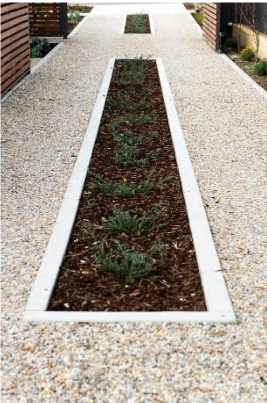
1C: The use of concrete kept to a minimum. Low carbon concrete used.
