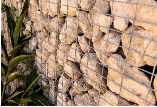
3B: Rubble rock walls and logs providing habitat for insects and lizards.
