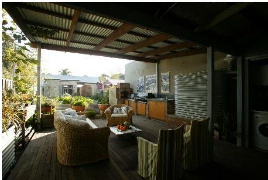
1B: Shading structure to northern side of house, angled to allow in winter light and provide summer shade.
