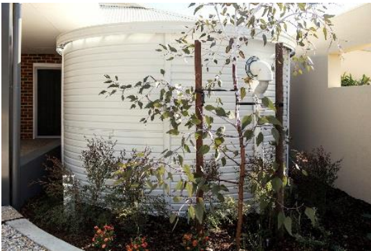
6D(i): Rainwater system – 20kL tank.
