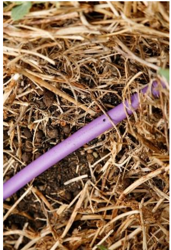
6B(iv): Greywater system – dripline.
