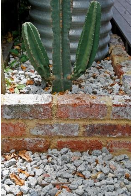
1A: Repurposed materials used where possible including timber, paving and aggregates.
