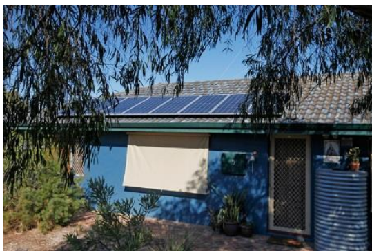
1A: Shading devices installed to exposed eastern and western facing windows.
