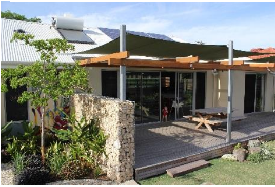
1A: Strategic positioning of trees, vines and shading devices for aiding thermal performance of the house.
