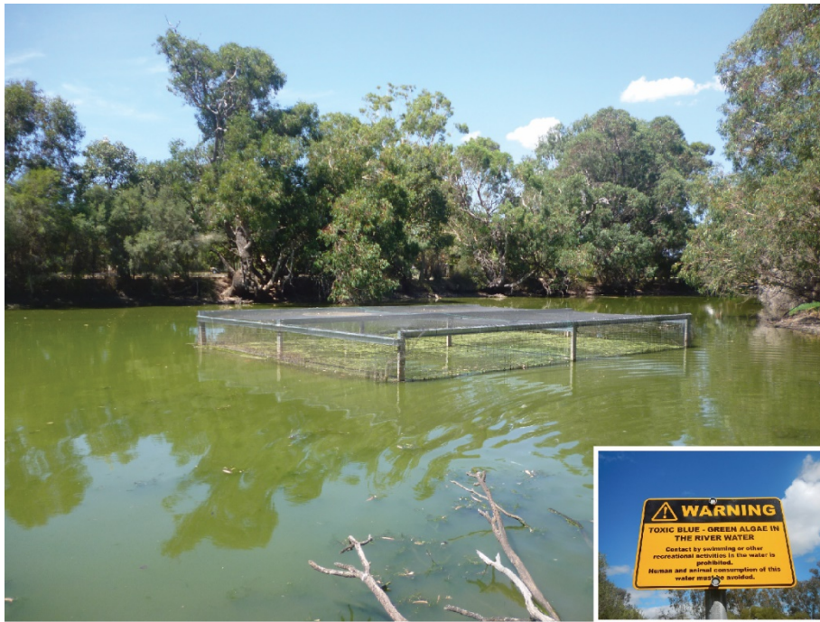
Figure 2.9. As a combined result of increased nutrient inputs, impoundment and flow diversion, the lower reach of the Vasse River experiences serious algal blooms each year during summer and autumn, closing the waters to public use. The structure in the river is an enclosure used in the restoration study (Chapter 5).
