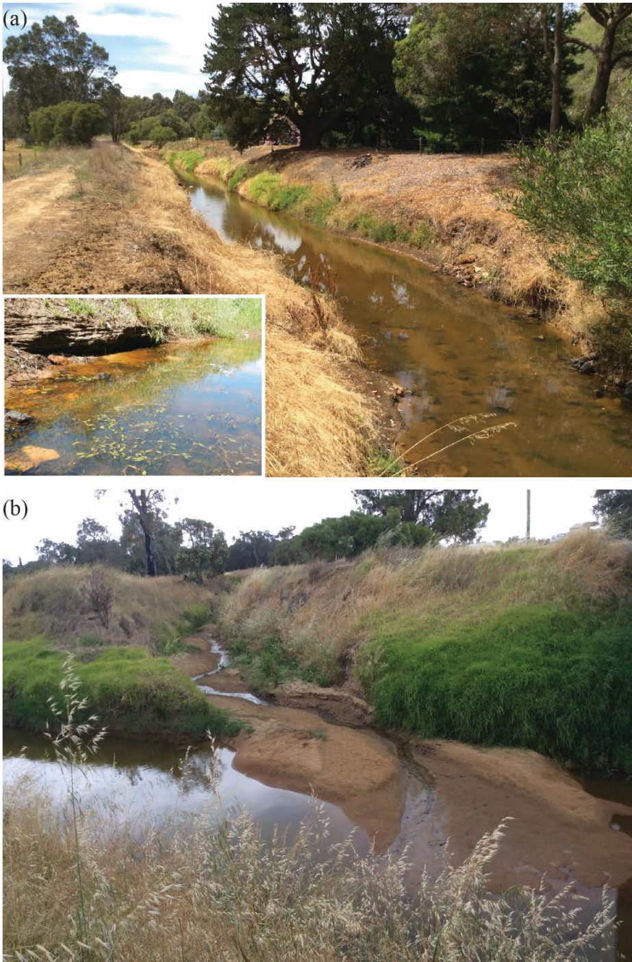
Figure 2.7. A tributary drain of the Buayanyup River (a) with no natural riparian vegetation, but which contains beds of Potamogeton drummondii and Ottelia ovalifolia , and another nearby tributary (b) showing bank slumping and severe sedimentation in the absence of riparian vegetation.
