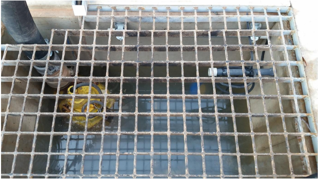
Figure 22: (Clampton, Site - Commission, 2015) – Sump pump (left), digital level switch (right). Tailings pit fills when the system overflows, the level switch activates the sump pump to recycle the water back into the tailings damn to be used again.
