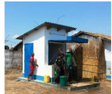
Figure 18: One of ten water kiosks in Ribáuè.
