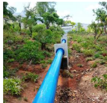
Figure 6: New pipeline from the reservoir into the town of Ribáuè.
