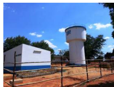
Figure 7: Rehabilitated uplifted water tank in the town centre.
