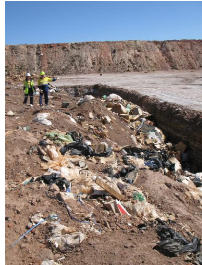
Figure 4.36: Cut & fill at RMS' landfill site
