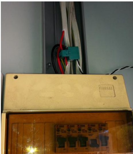
Figure 3.22 Current transformer
