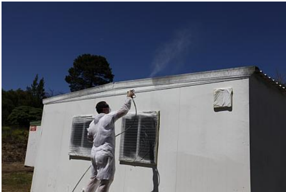
Figure 3.21: Primer coating being applied.
