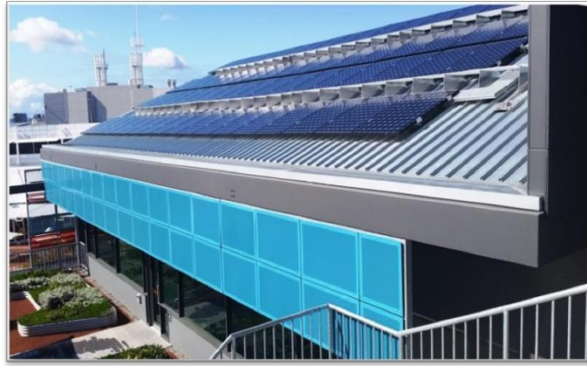
Figure 3. Roof Solar PV.
