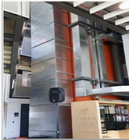
Figure 2. Exposed structural steel and building elements.
