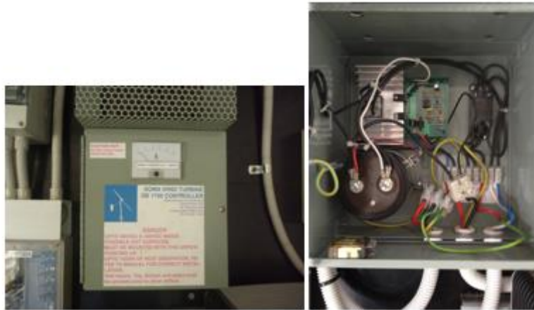
Figure 8- Controller Connections
