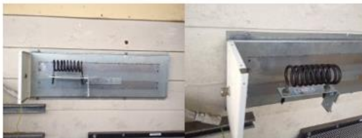
Figure 9-Bracket Made to Hold Dump Resistor
