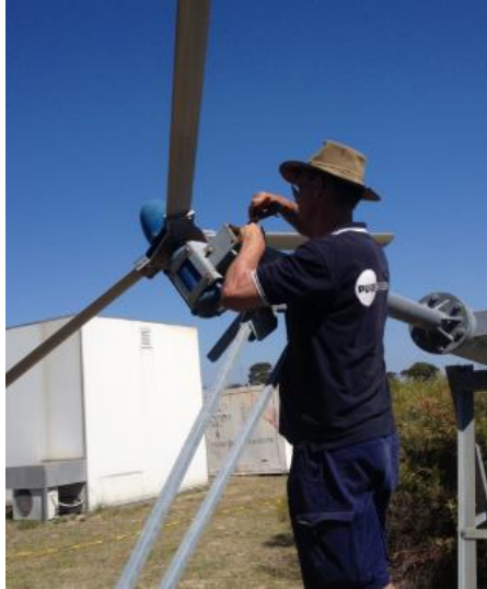
Figure 29- Opening to check slip rings
