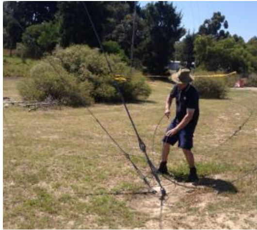
Figure 22-Side guys and Gin pole side stray wires always have slack
