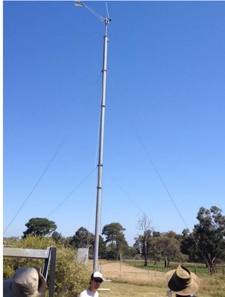
Figure 18- FP Turbine Upright position
