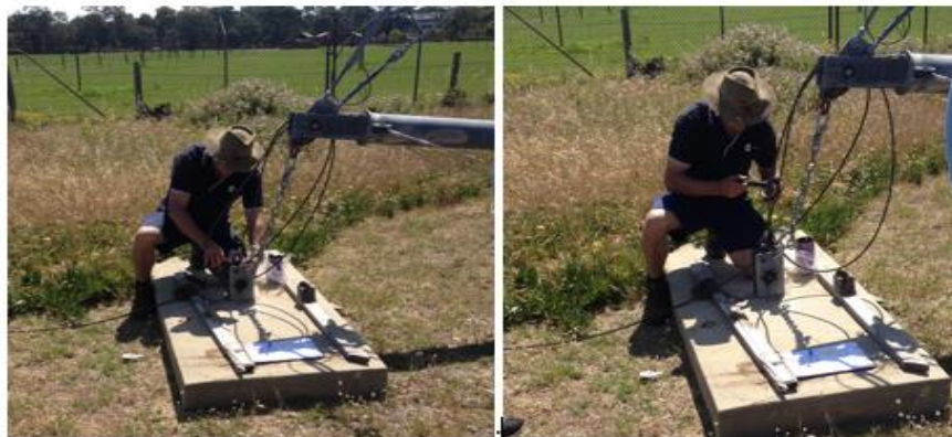
Figure 19- Attached Pullies and cable to gin pole
