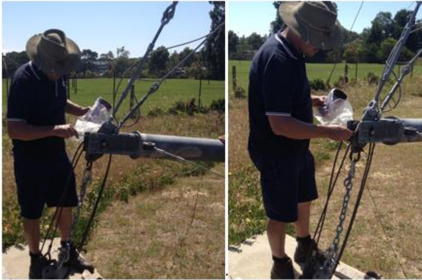
Figure 20-Apply grease to the cable
