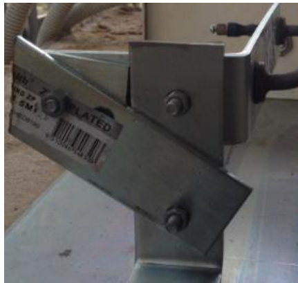
Figure 9-Bracket Made to Hold Dump Resistor
