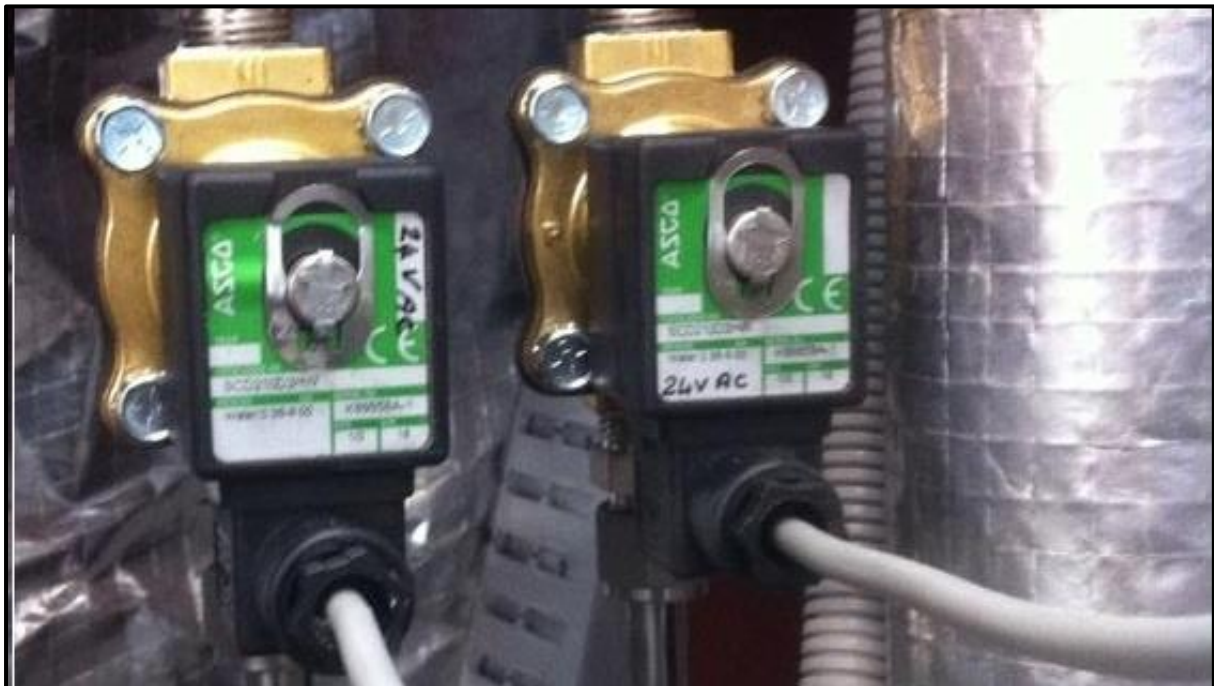
Figure 37: SV Raw Water and Control Air
