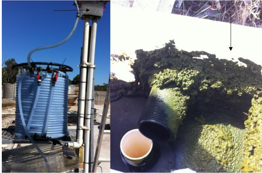
Figure 6. Cells sticking and accumulating inside the Biocoil in the degasser box
