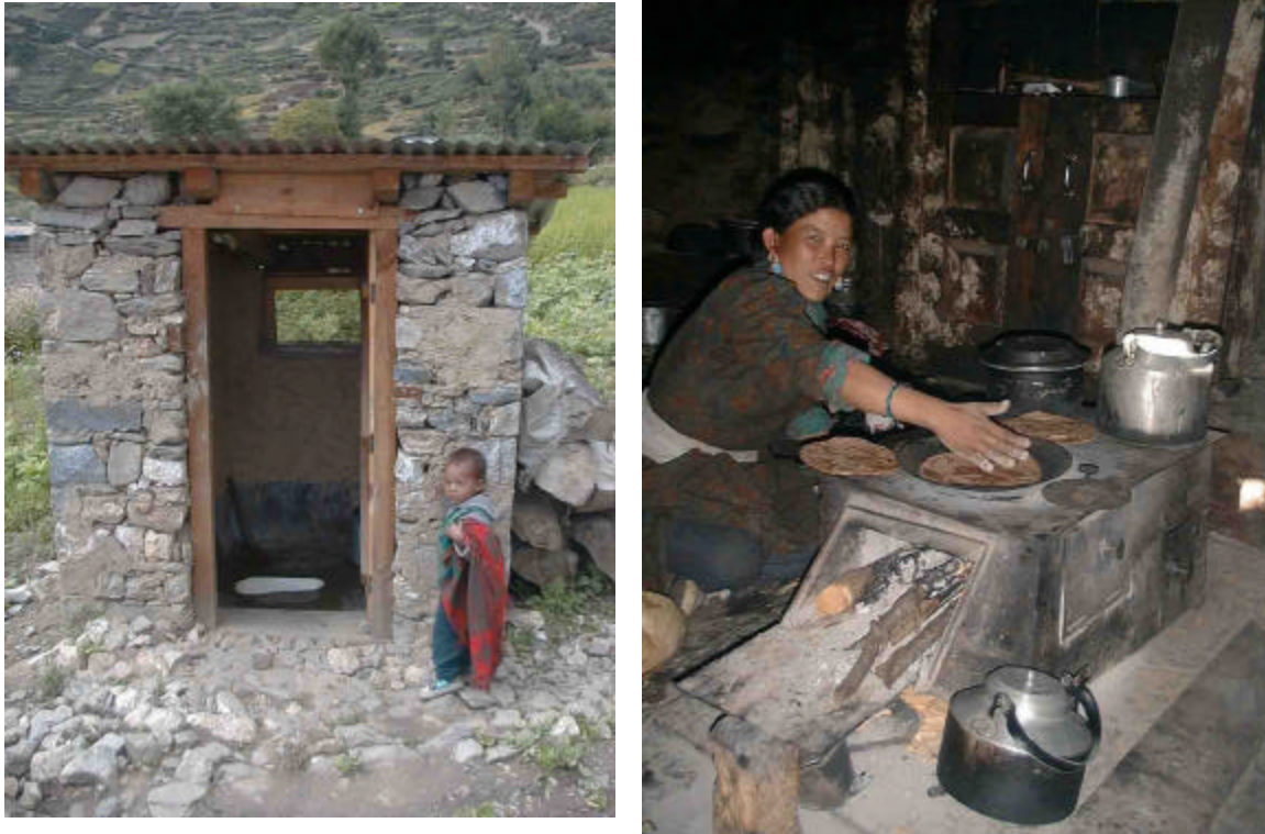
Figure 4. Left: pit latrine built to obtain stove subsidy. Right: smokeless stove – but it is difficult to persuade people to close the door to increase the efficiency.
