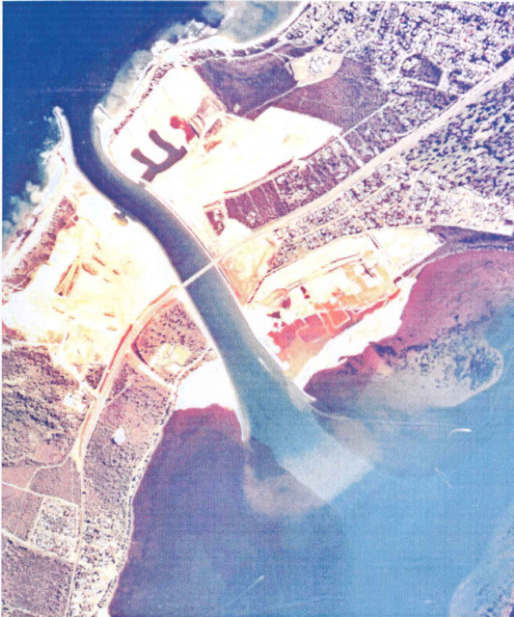
Figure 1.2: Aerial photograph of the Dawesville channel. Channel dimensions are 200 m wide and 4.5 m (AHD) deep at the junction of the estuary, tapering to 150 m wide and 6.5 m deep at Indian Ocean entrance (Kinhill, 1988).
