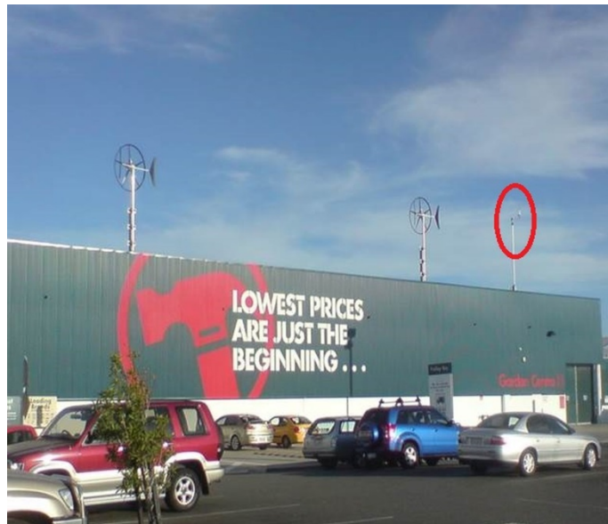
Figure 2. A photograph of the front view of the Bunnings warehouse showing the five small wind turbines and the ultrasonic anemometer position (red circle).
