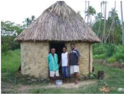
Figure 2.2.3h. View thatch walls using local bamboo fibre, harvested and woven.
