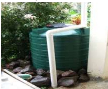
Figure 2.2.3o. We added a 500l rainwater water tank; diverted from roof gutters; on local rock foundation; and made a rock frog pond with the overflow system.
