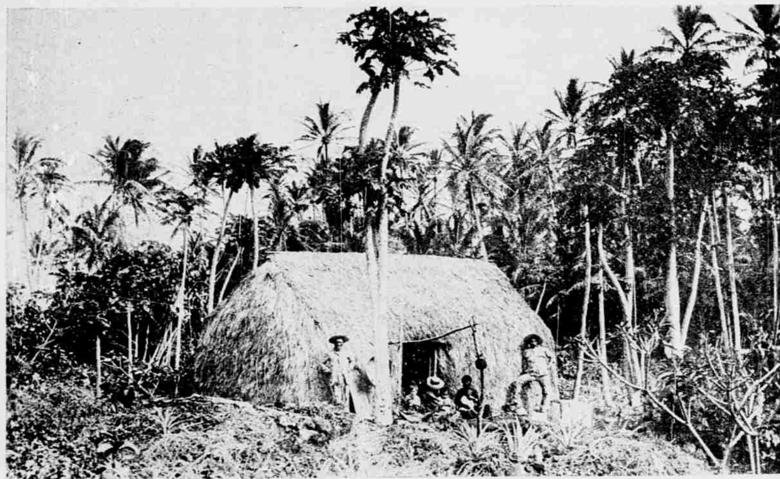
A PUNA RESIDENCE ON THE LINE OF THE HILO RAILROAD.
