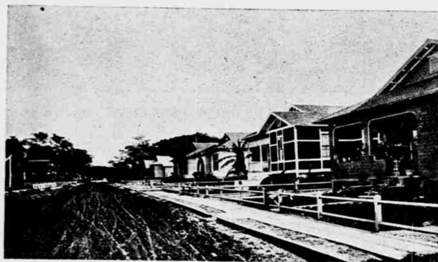
MATLOCK AVENUE—CAMPBELL COTTAGES.
