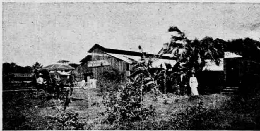
W. H. CAMPBELL'S Mill and Office.
