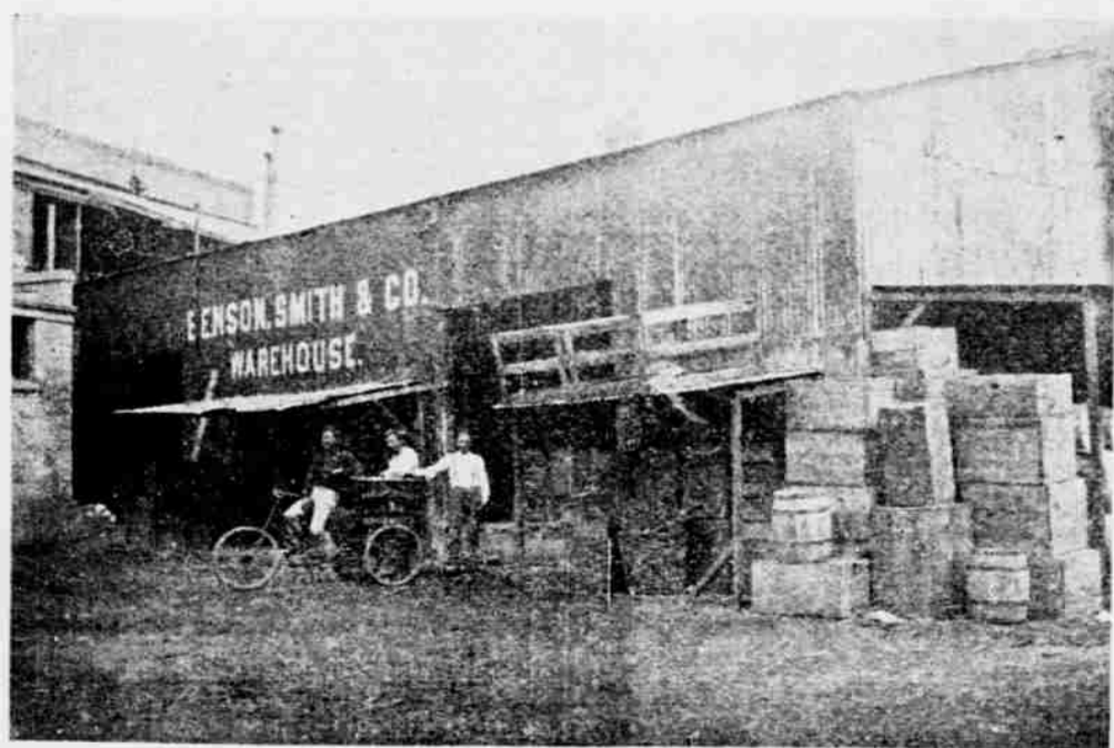
BENSON SMITH &amp; CO., WAREHOUSE.
