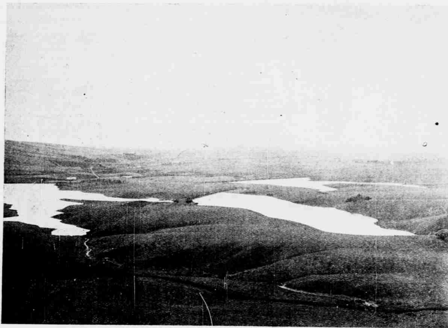
Group of Storage Reservoirs on McBryde Plantation for storm water covering 48.30 acres. Elevation above sea level 650 feet. Combined capacity 300,000,000 gallons.
