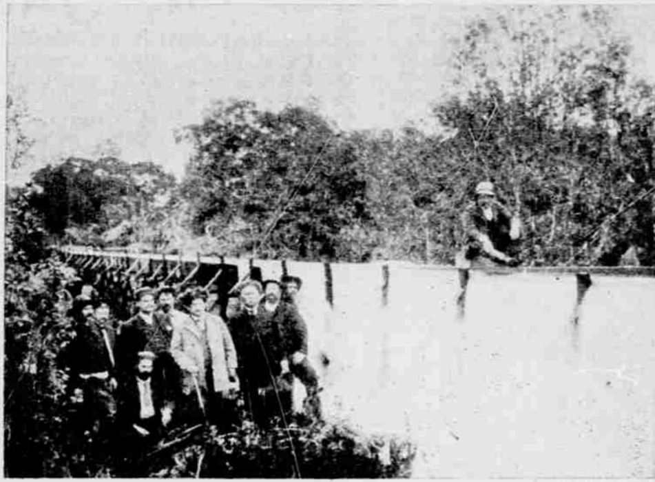
OLAA WATER FLUME.
