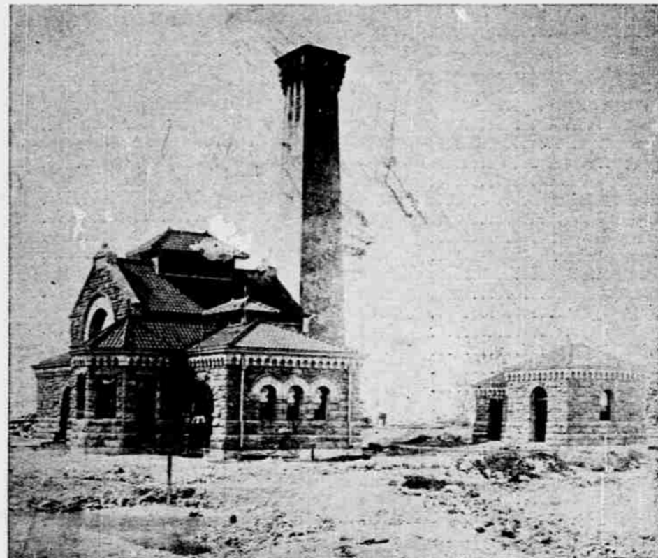
SEWER PUMPING STATION.
