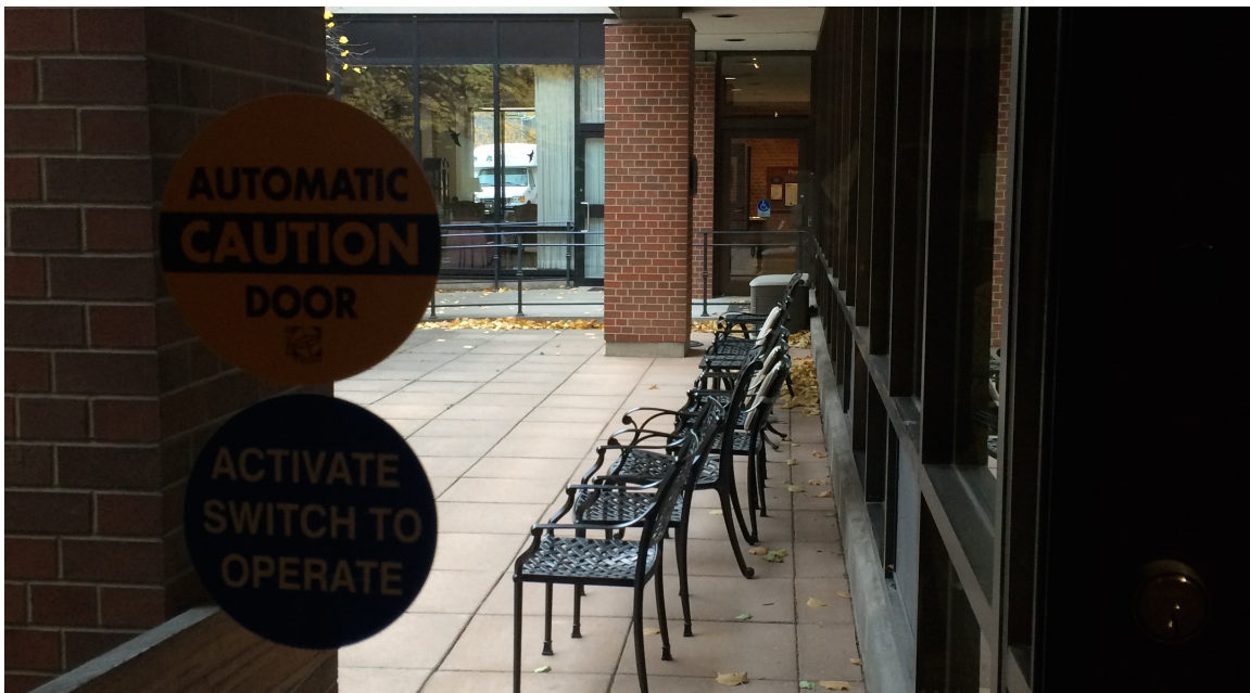
Figure 8: Belmont House Egress to Garden
