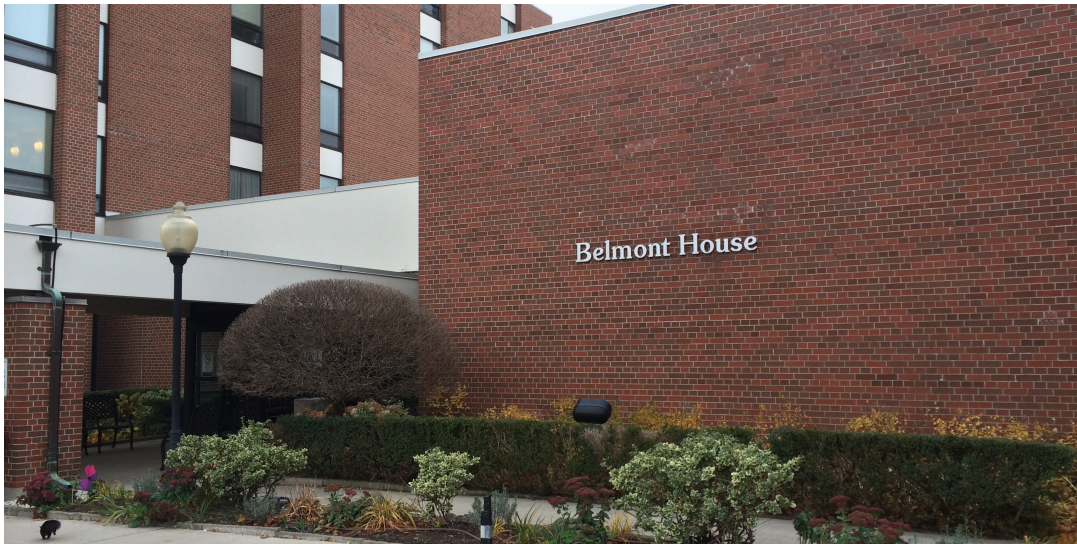
Figure 6: Belmont House Exterior
