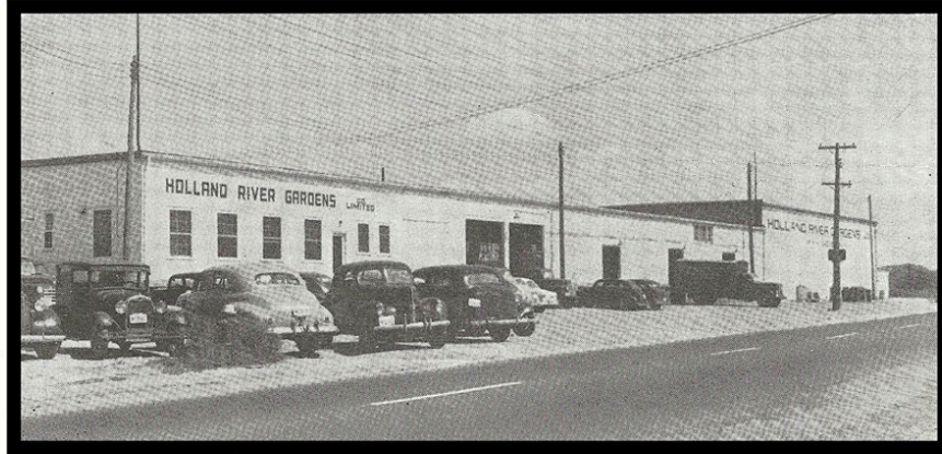
A VIEW OF HOLLAND RIVER GARDENS CO. LIMITED'S ICE-PACKING PLANT, APPROACHING FROM THE NORTH.
