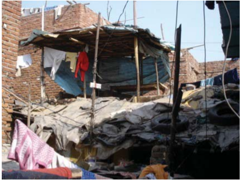
Figure 1: A house in NOIDA shanty settlement, with brick walls and a tarpaulin roof held up by bamboo sticks.
