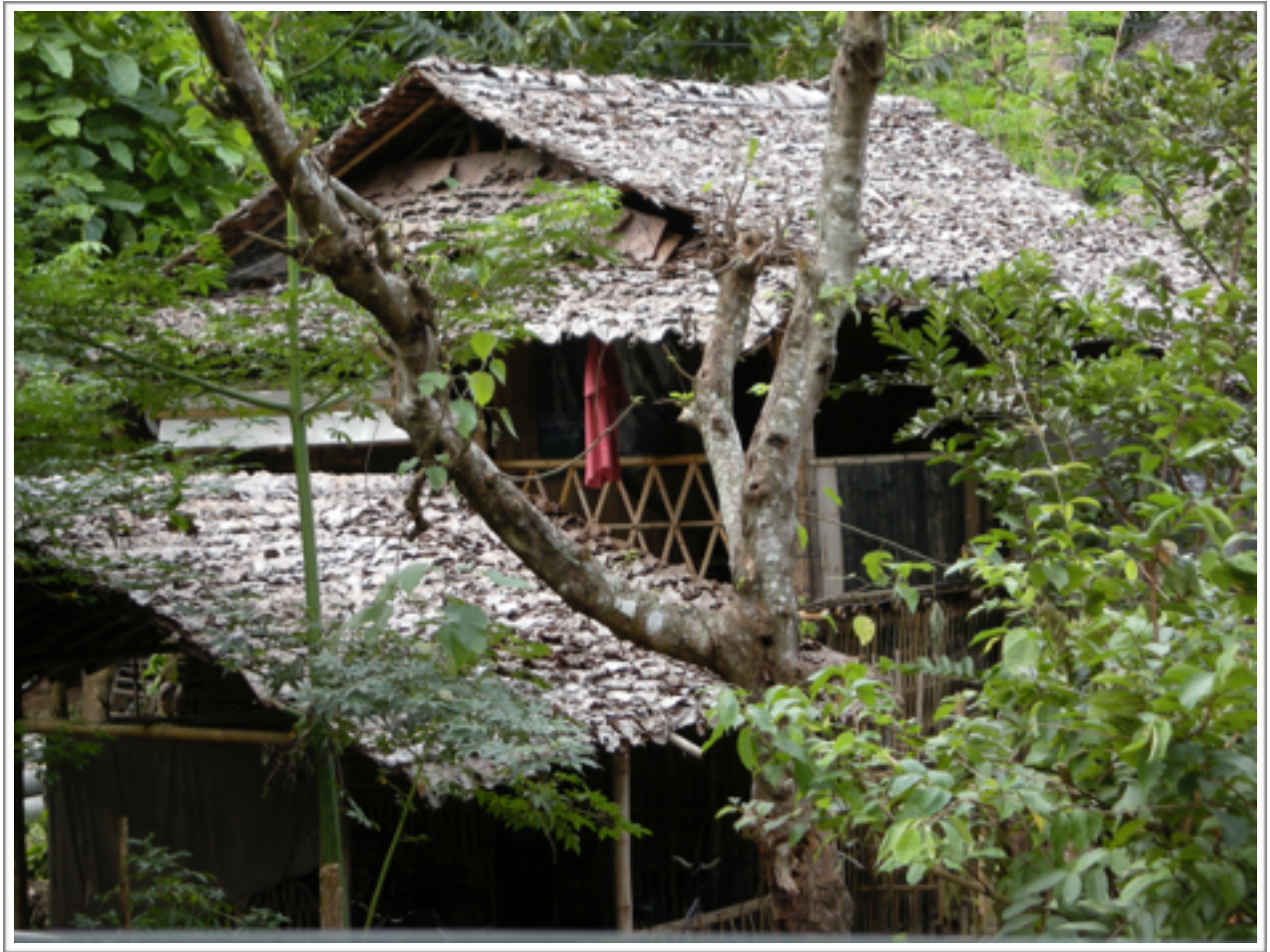
Figure 5.1. A house at Mae La camp fashioned of wood and bamboo for the main structure and leaves for the roof in Section A.
