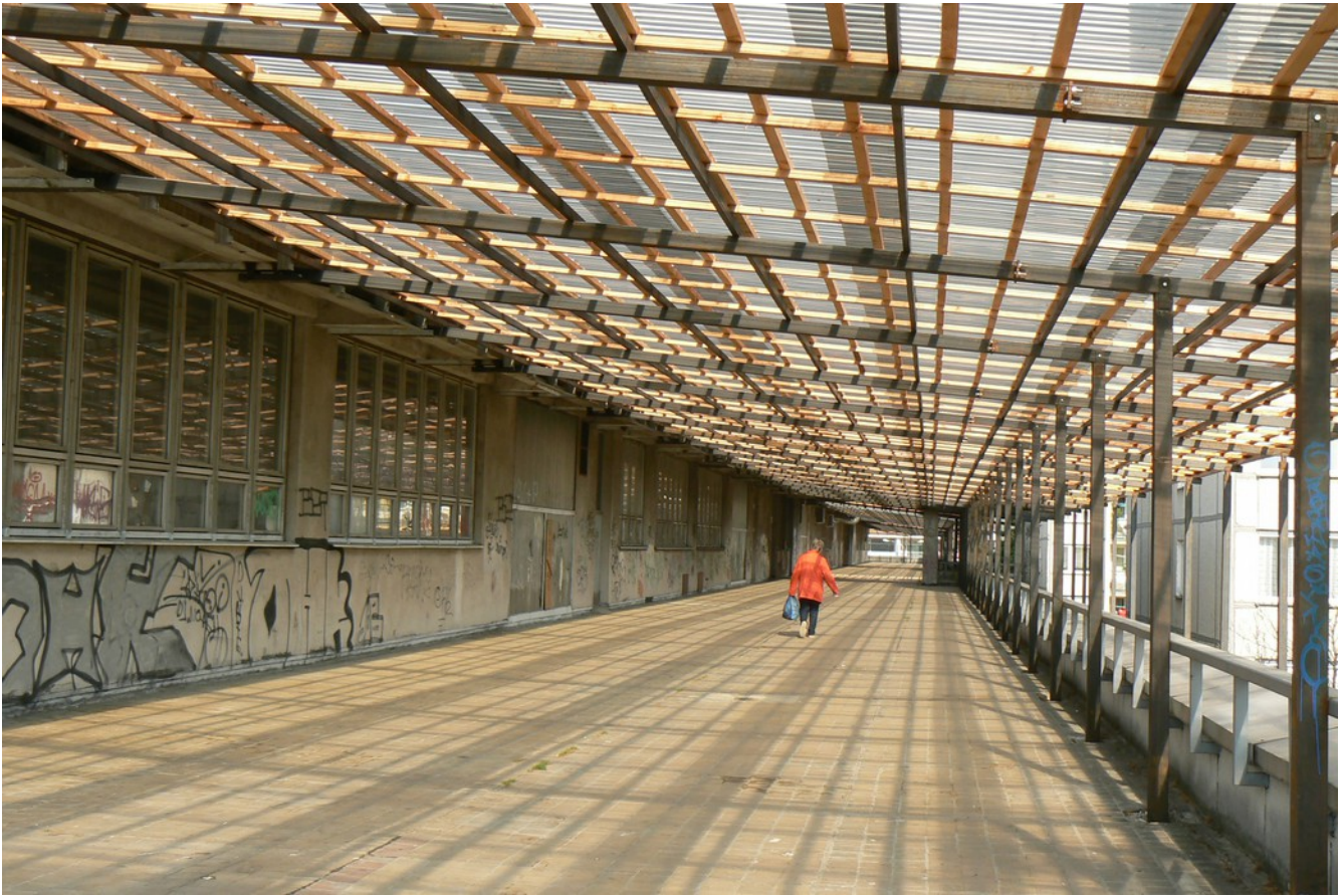
Fig. 5.11. Pedestrian walkway. Part of South City's anaesthetic pedestrian landscape.
