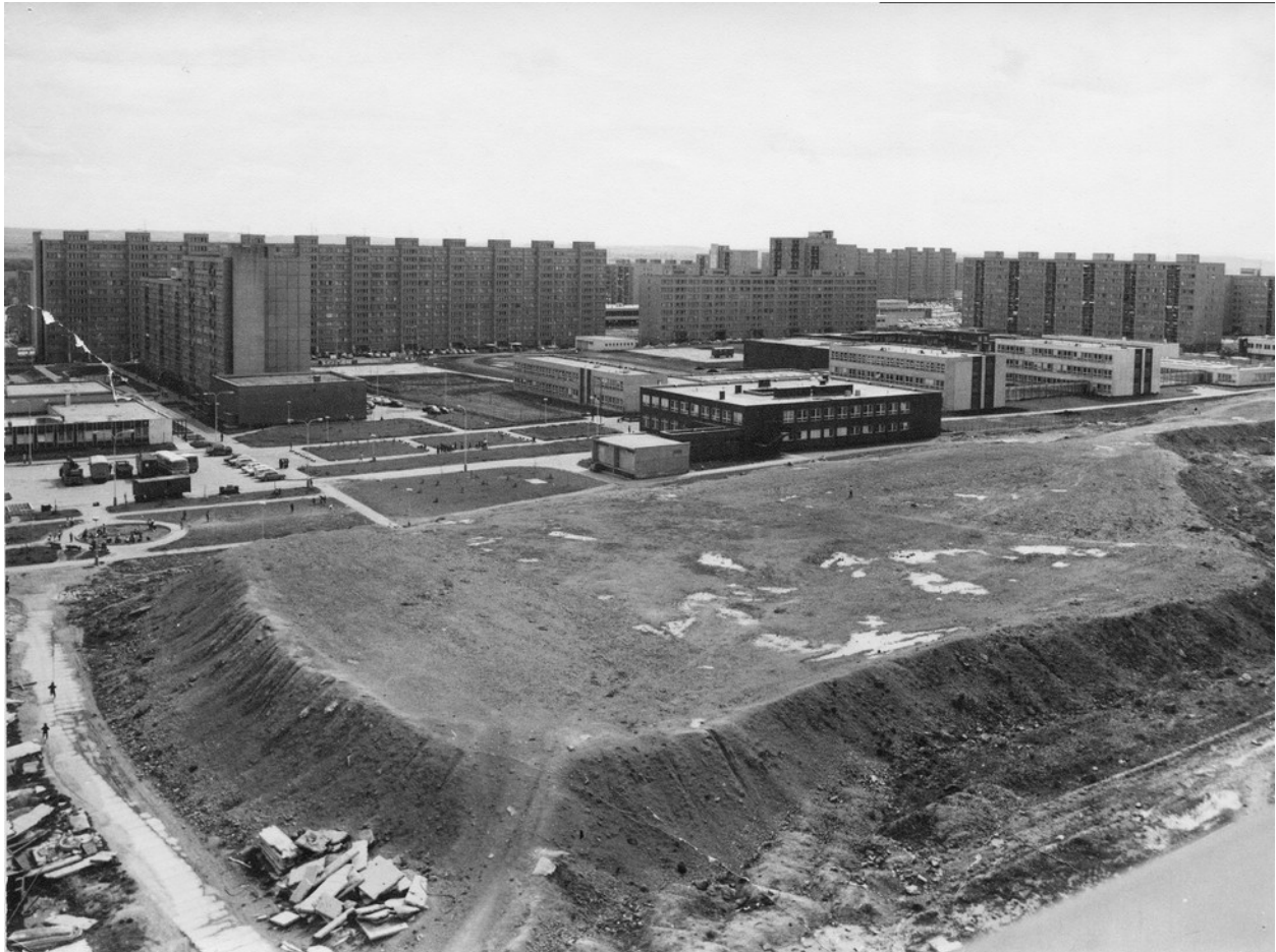
Fig. 5.8. The mound of excavated earth sitting in what would become South City's Central Park. (Courtesy of Jiří Lasovský.)
