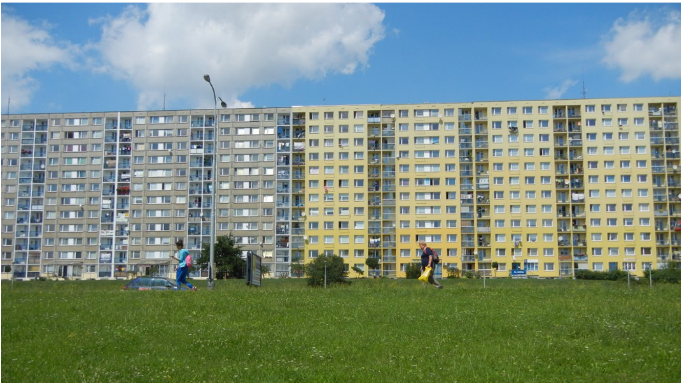
Fig. 5.12. Contrasting facades in South City. This picture is taken from a field where one of South City's local centres was to be built.
