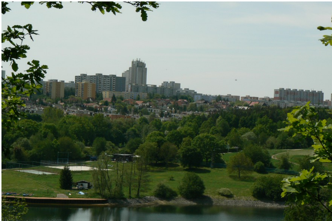
Fig. 5.16. South City seen from the east in the Hostivař recreational area. The family houses of South City as well as houses from the previous settlement can be seen just beyond the trees.
