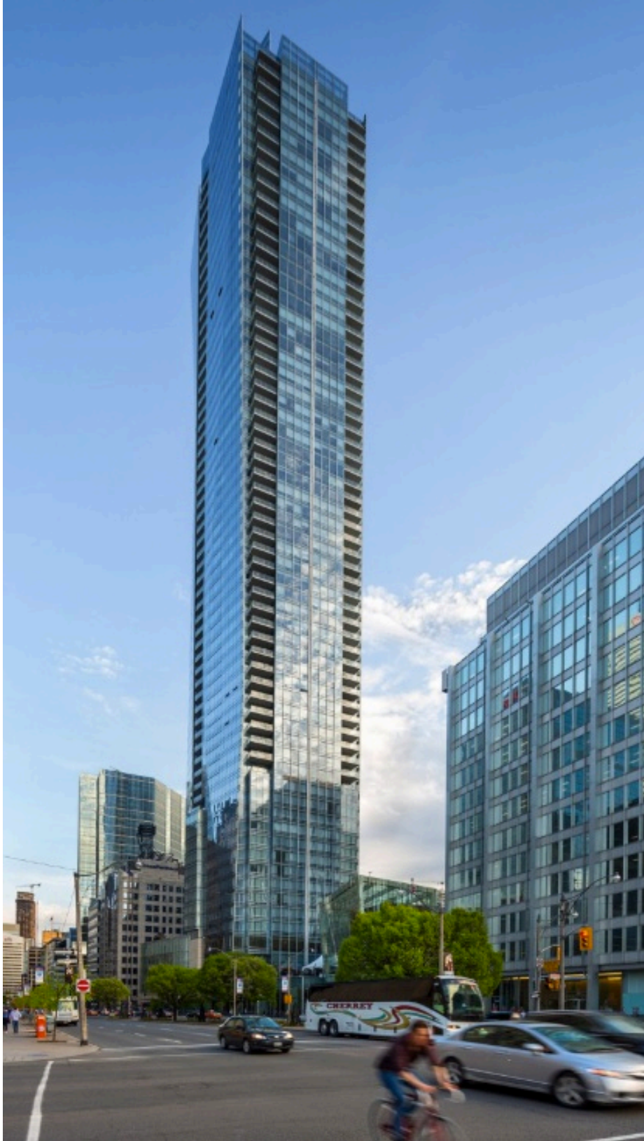
Above: Shangri-La, looking southward from Queen & University. Source: westbankcorp.com
