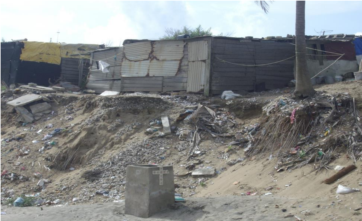
Figure 30. Coastal erosion impacts on housing.
