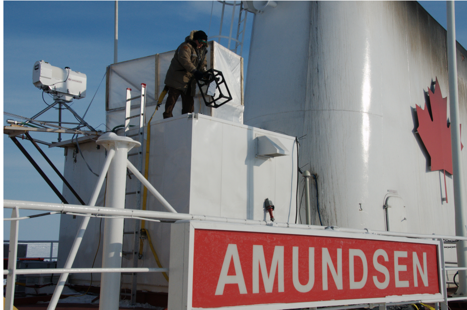
(a) Installation of the external mirror to the top of the laboratory container. The external mirror was used to direct the lidar field of view to 10^\circ above horizontal.
