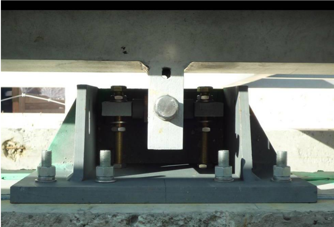
Figure C.16. Adjustable panel bracket (Courtesy of © Marc Simmons, 2015)
