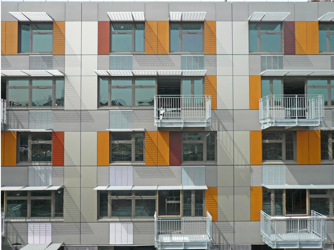
Figure B.2. Balcony doors between mega panels (Courtesy of © Marc Simmons, 2015)
