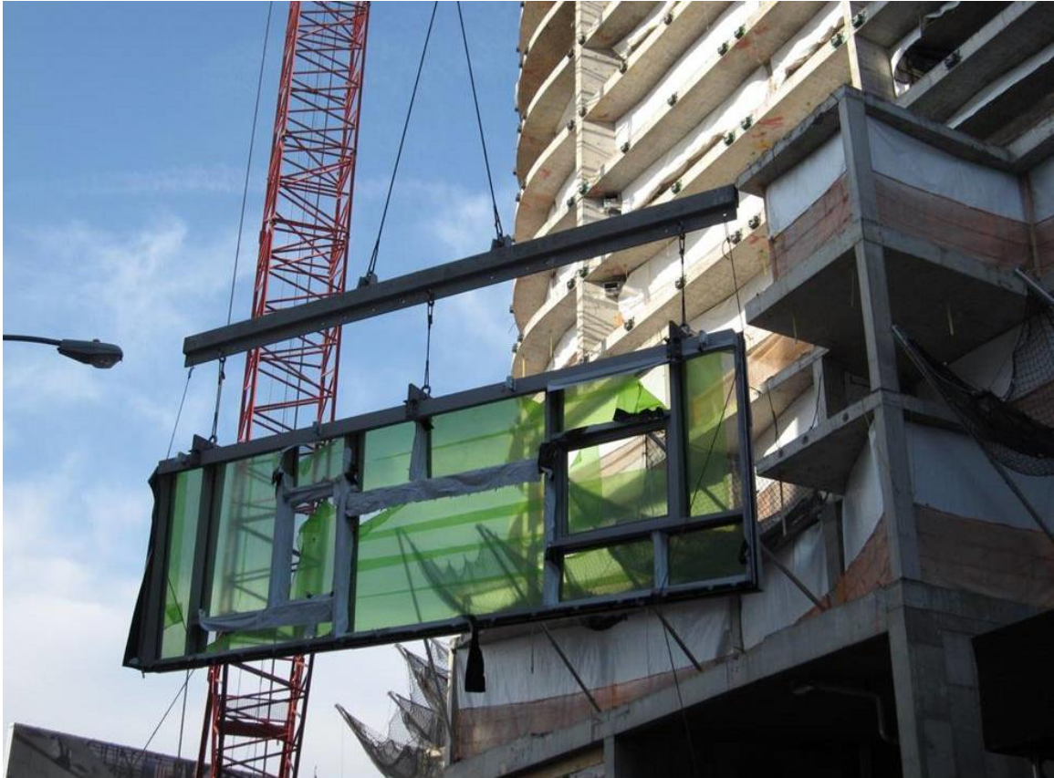
Figure C.8. Crane lifting the prefab panel (Courtesy of © Marc Simmons, 2015)
