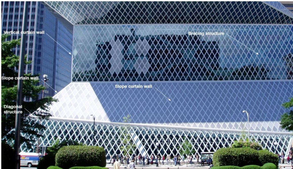
Figure 4.8. Case study one, sub-assemblies of the diagrid façade (Courtesy of © Marc Simmons, 2015)
