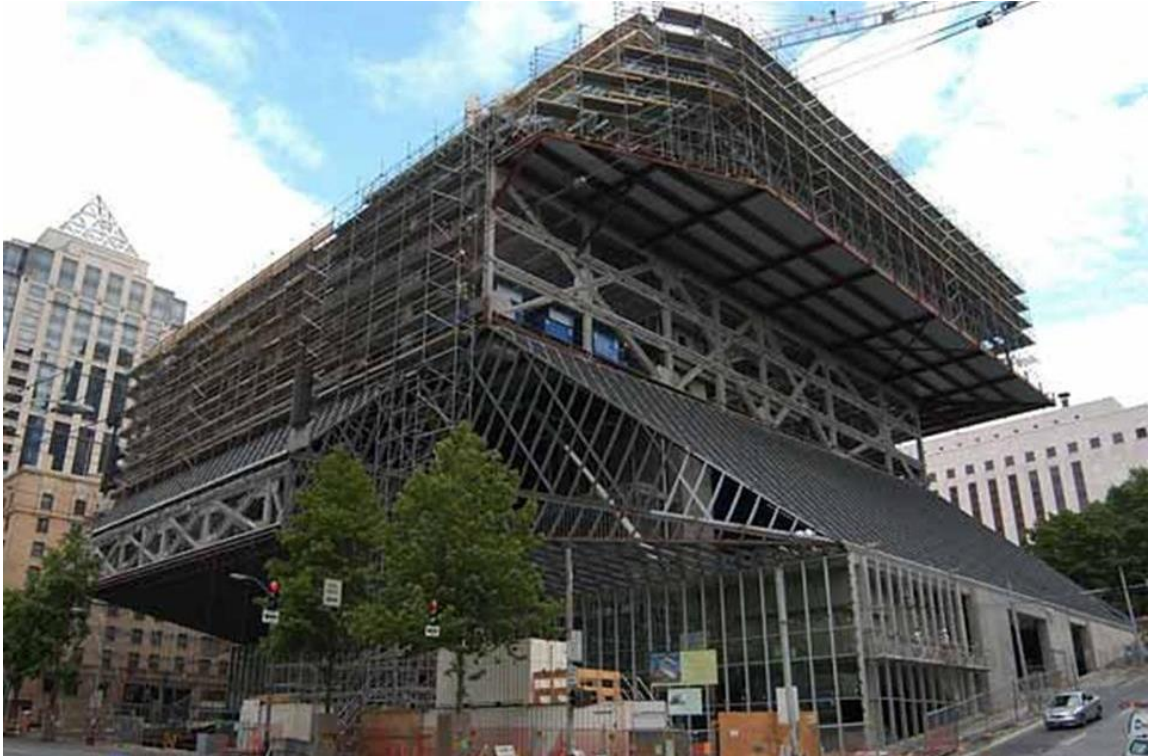
Figure A.13. Façade differentiation according to structural requirements (Courtesy of © Marc Simmons, 2015)
