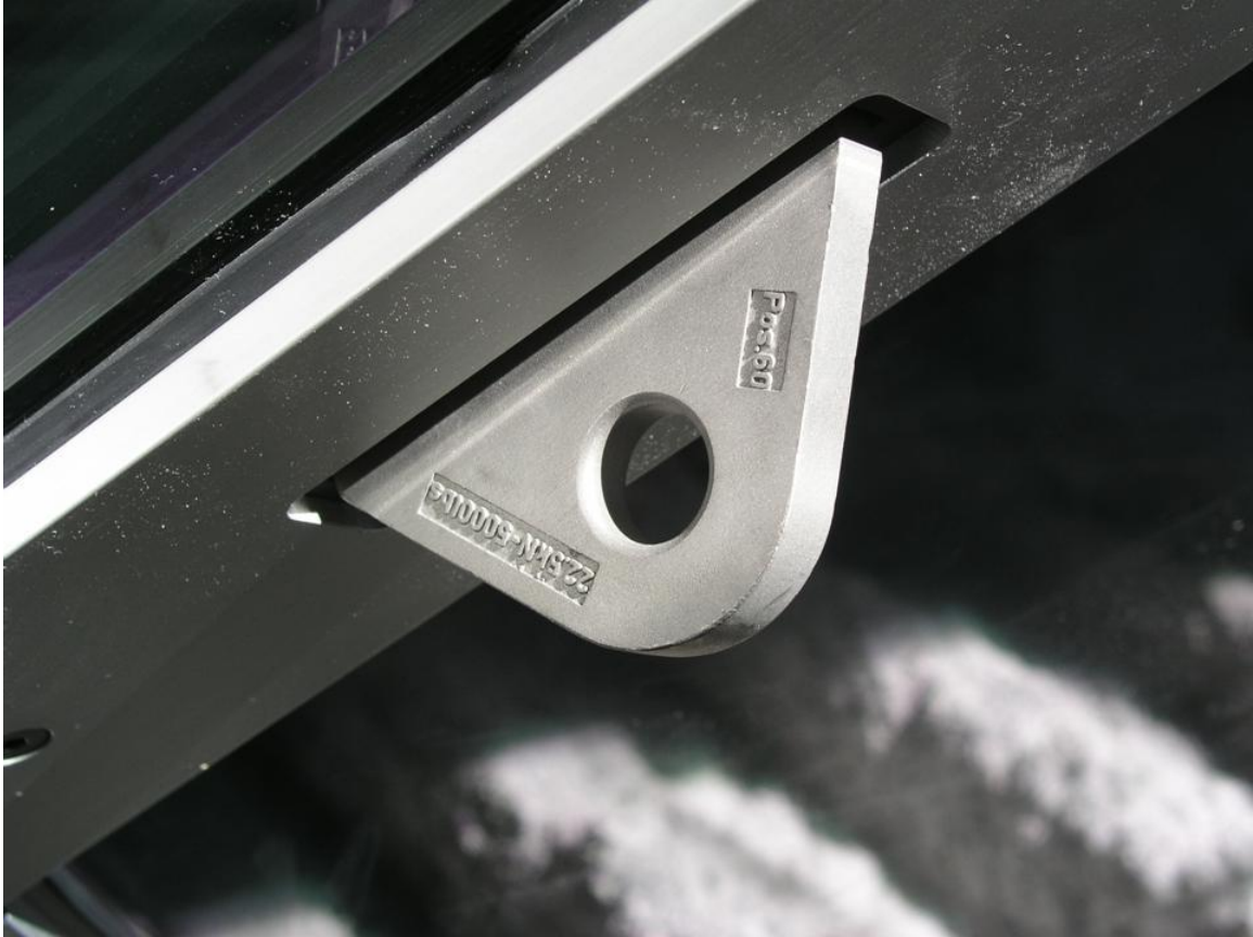
Figure A.9. Connection blade that supports the cleaning crew (Courtesy of © Marc Simmons, 2015)
