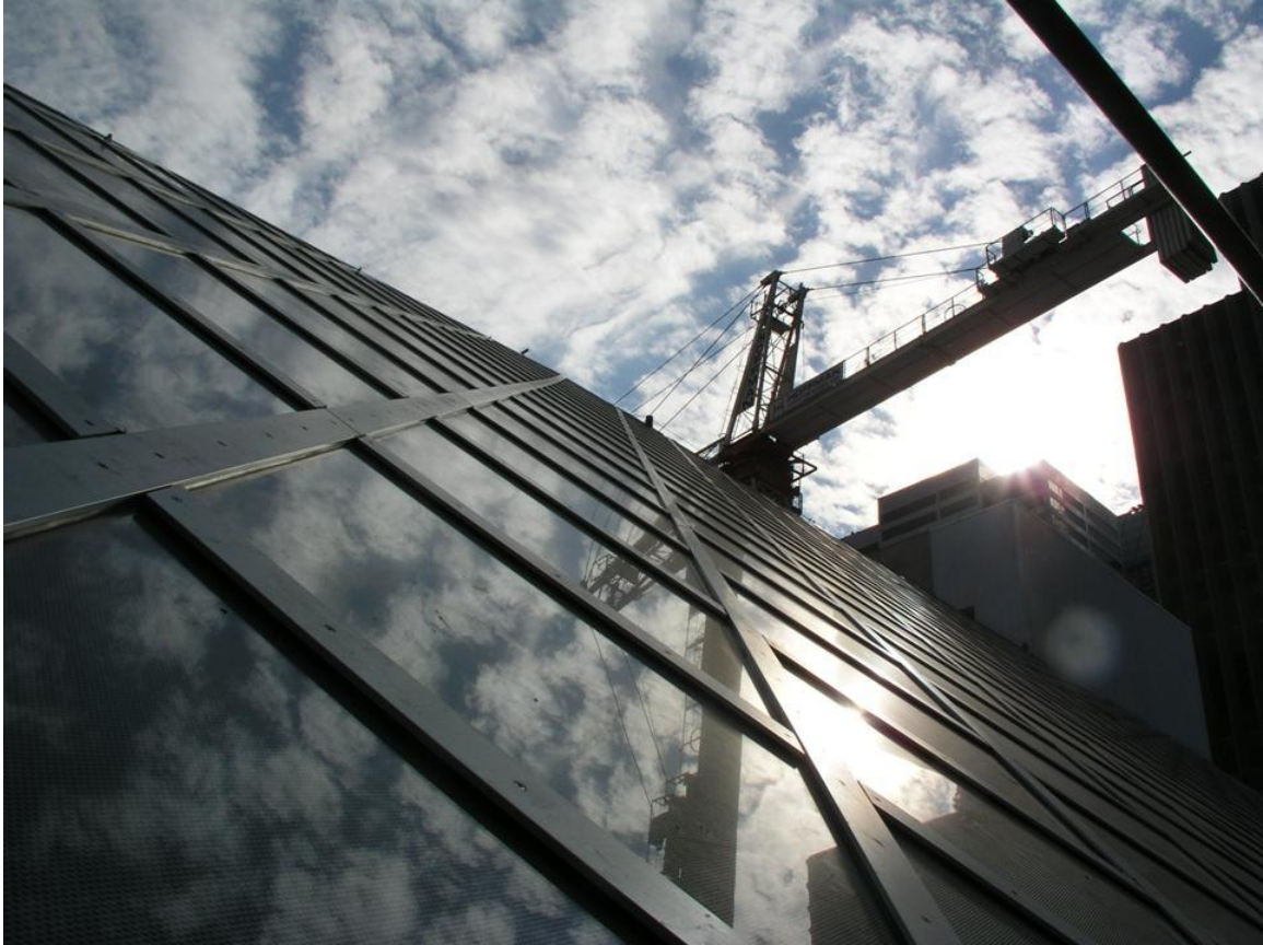
Figure A.17. Façade surface cap holding glass panels (Courtesy of © Marc Simmons, 2015)
