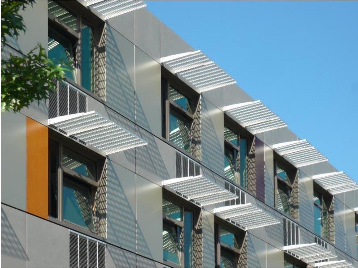
Figure B.5. Mega panels brise-soleils (Courtesy of © Marc Simmons, 2015)
