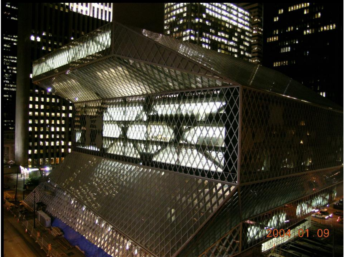
Figure 4.2. Façade regions sharing the same diagrid pattern (Courtesy of © Marc Simmons, 2015)
