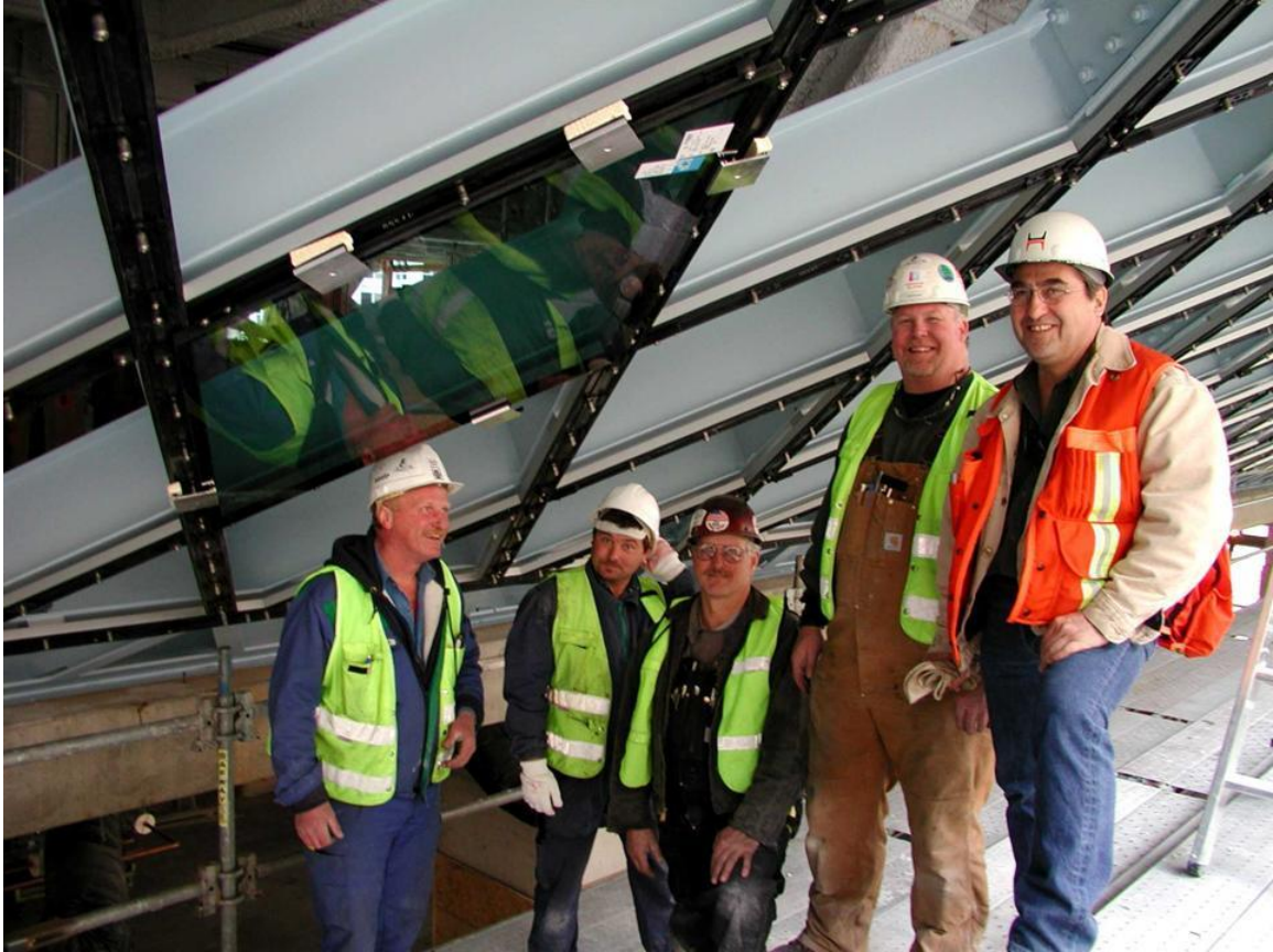
Figure A.19, Glass installation (Courtesy of © Marc Simmons, 2015)
