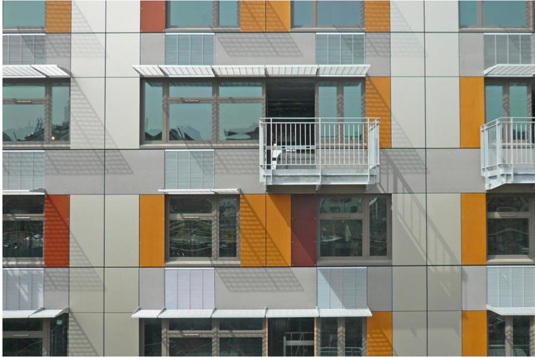
Figure 4.3. Via Verde mega panels (Courtesy of © Marc Simmons, 2015)
