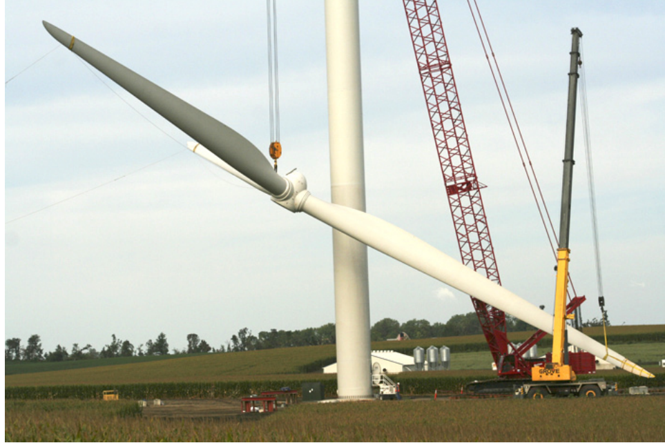
Figure 1.1: Erection of Wind Turbine 1
