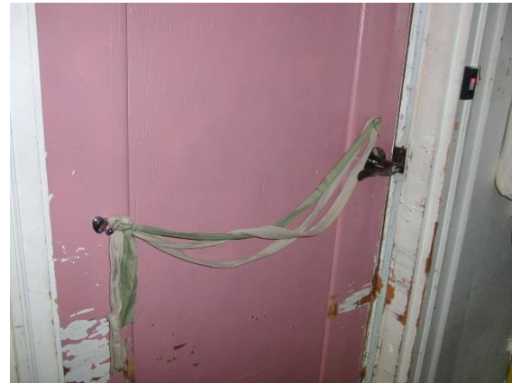
Figure 1. Example of a homemade door pull. Damage from the user's wheelchair to the doorframe can also be seen.
