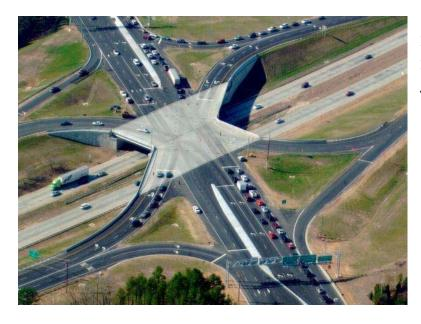
Figure 32. Example of SPUI form from I-40 in Durham, NC *Source: Esawey & Sayed 2012*
