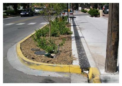
extension and the curb as opposed to one solid piece. This small canal allows storm water to drain past the extension and not create an unsafe build-up at the intersection.
