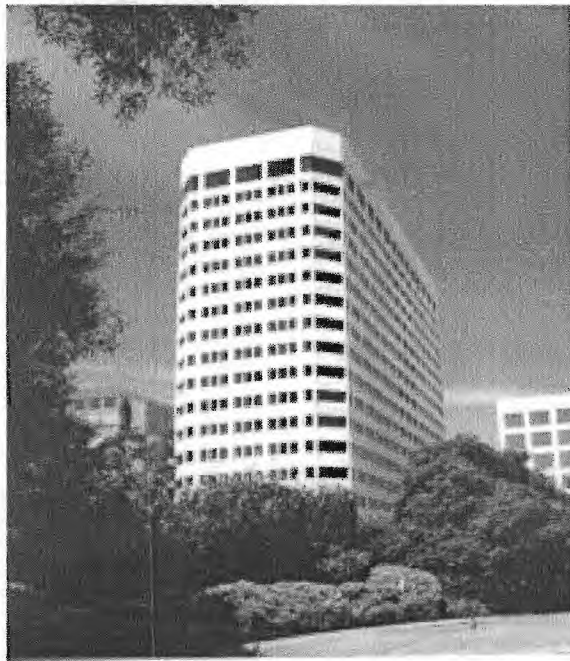
Figure 4.1 : Baseline Building on West Coast of U.S.
