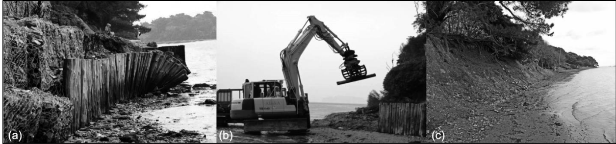
Figure 2. (a) Failing coastal protection structures in Brownsea Island (b) were removed in 2011 and (c) by 2013 the shore profile was similar to pre-protection times (Photos: Tony Flux).
