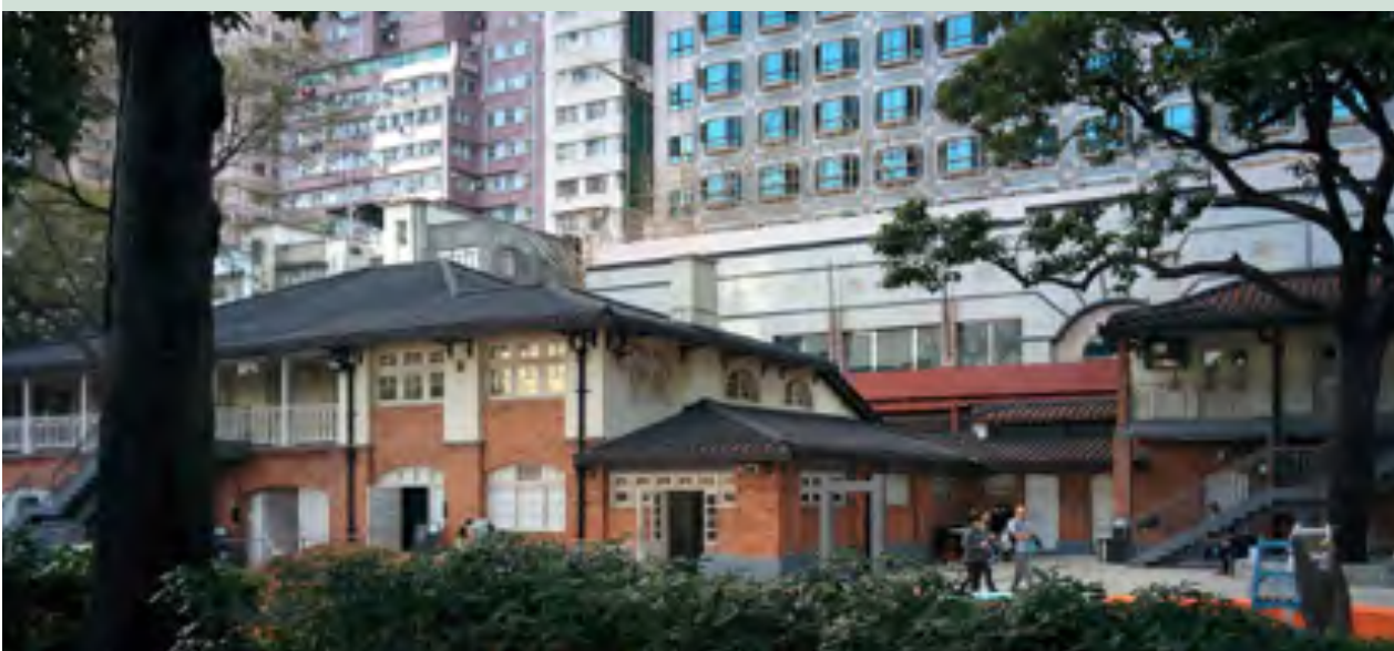
Image 1: The historical building was transformed into an art space "Oi!" committed to community art
