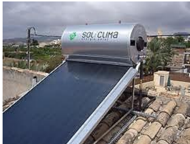
Figure 1-9 Thermo-syphon for domestic applications [19]
