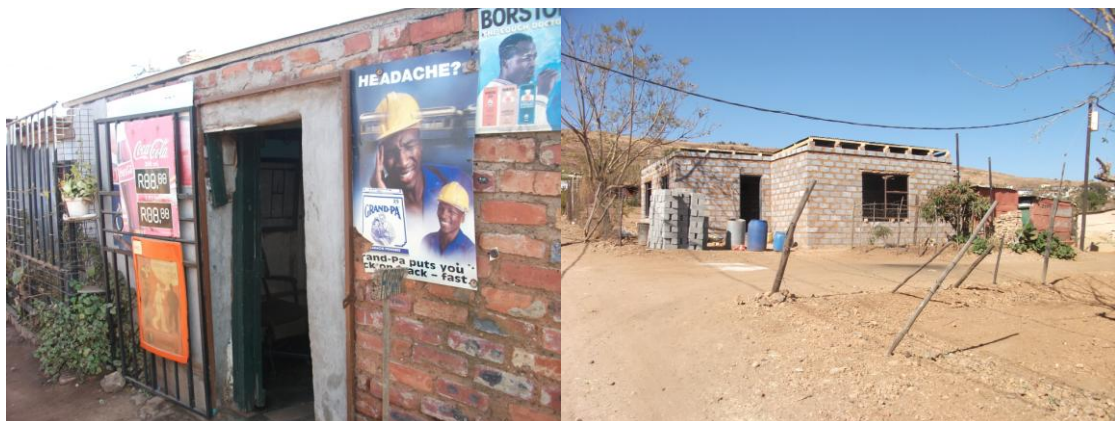
Brick constructions in Jeffsville (left) and Brazzaville (right)
